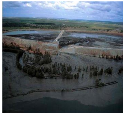
Figure 5. Los Frailes tailings failure (Ref http://en.wikipedia.org/wiki/Dam_failure )
