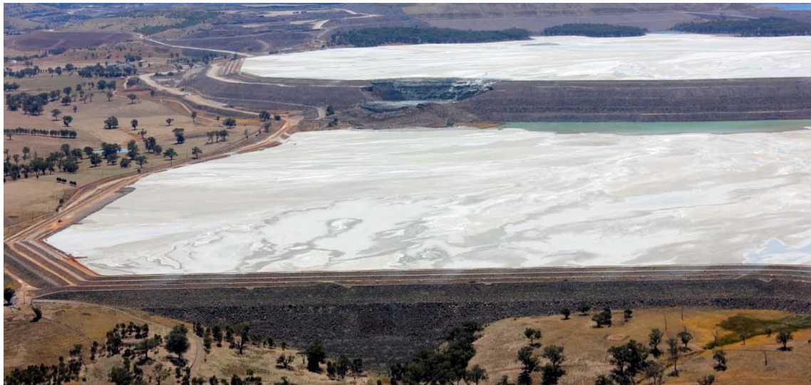
Figure 3. Slope failure in upper compartment at Cadia, Australia (Cadia press release, 2018)
